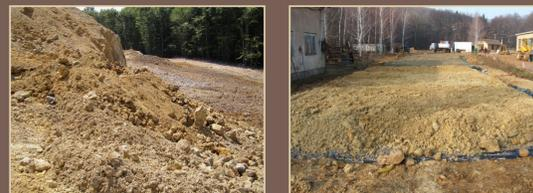
Fig. 3. and 4. The Bányabérc mine waste heap under excavation near the Bányabérc shaft and the field plots constructed from BB mine waste.
